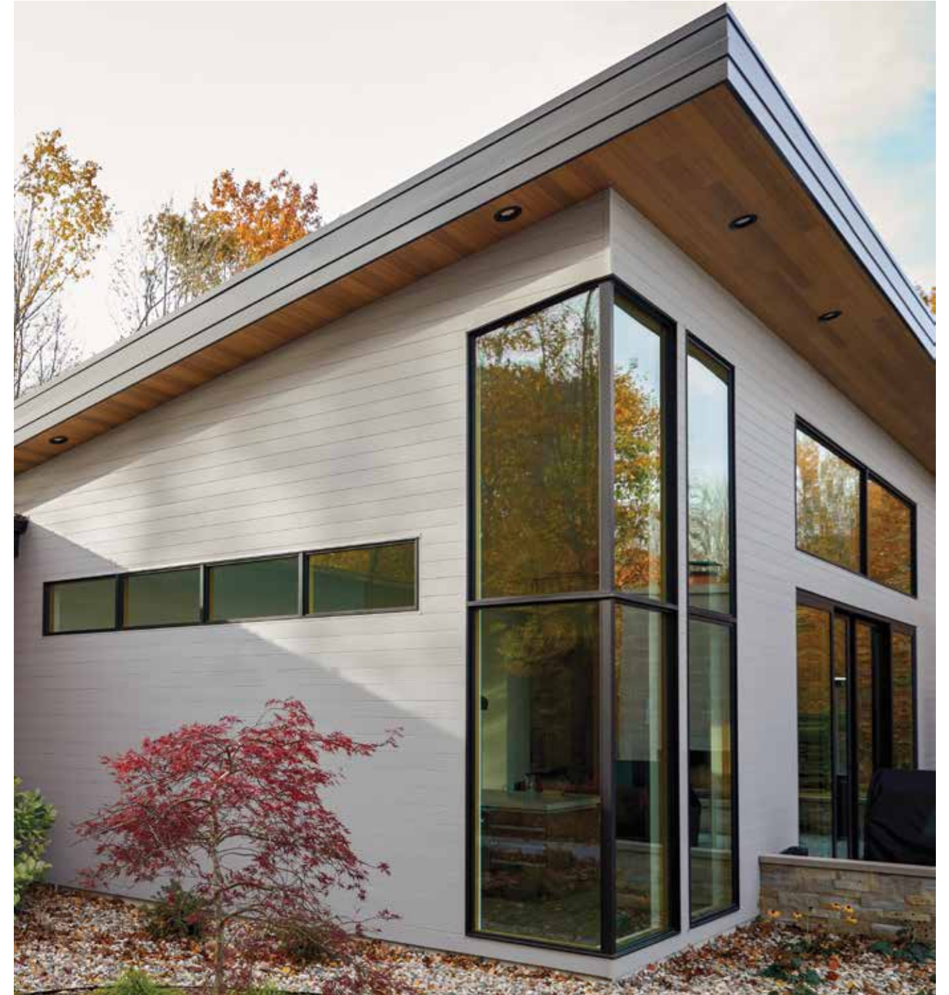
462 Silver Lining [SVRL] 5" Plank Horizontal Siding and 482 Gilded Grain [GILD] 5" Plank Soffit
